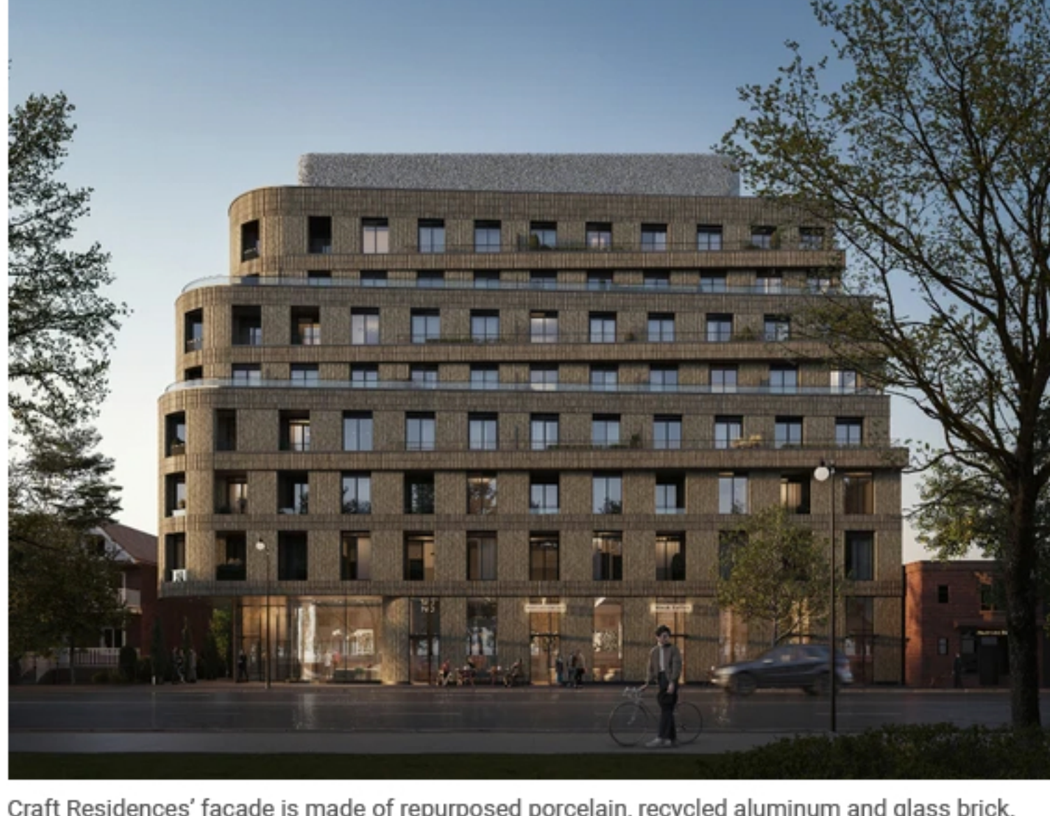
Craft Residences' façade is made of repurposed porcelain, recycled aluminum and glass brick. PHOTO BY PHOTO COURTESY OF JORG
